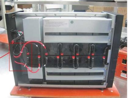
**Note: Tie cables together** So you finish assembling batteries and you can fix the cover now.
